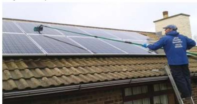
Figure : A person cleaning PV panels manually with water fed pole.
